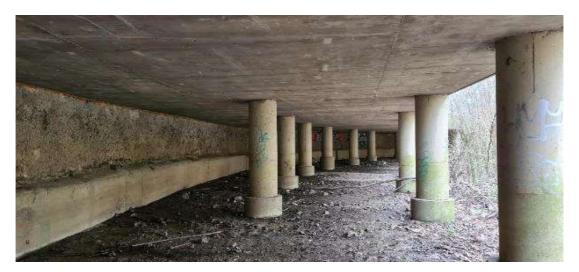
Figure 13: View from the stilt structure supporting Longbridge SLTL
