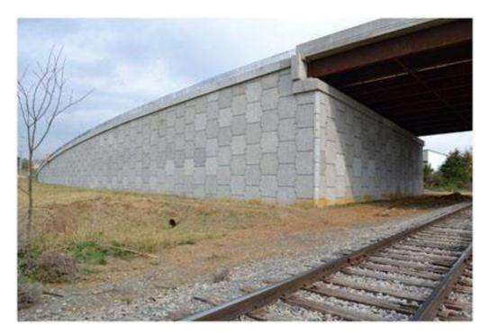
Figure 26: Typical concrete faced reinforced earth retaining wall (Example by RECo®)
